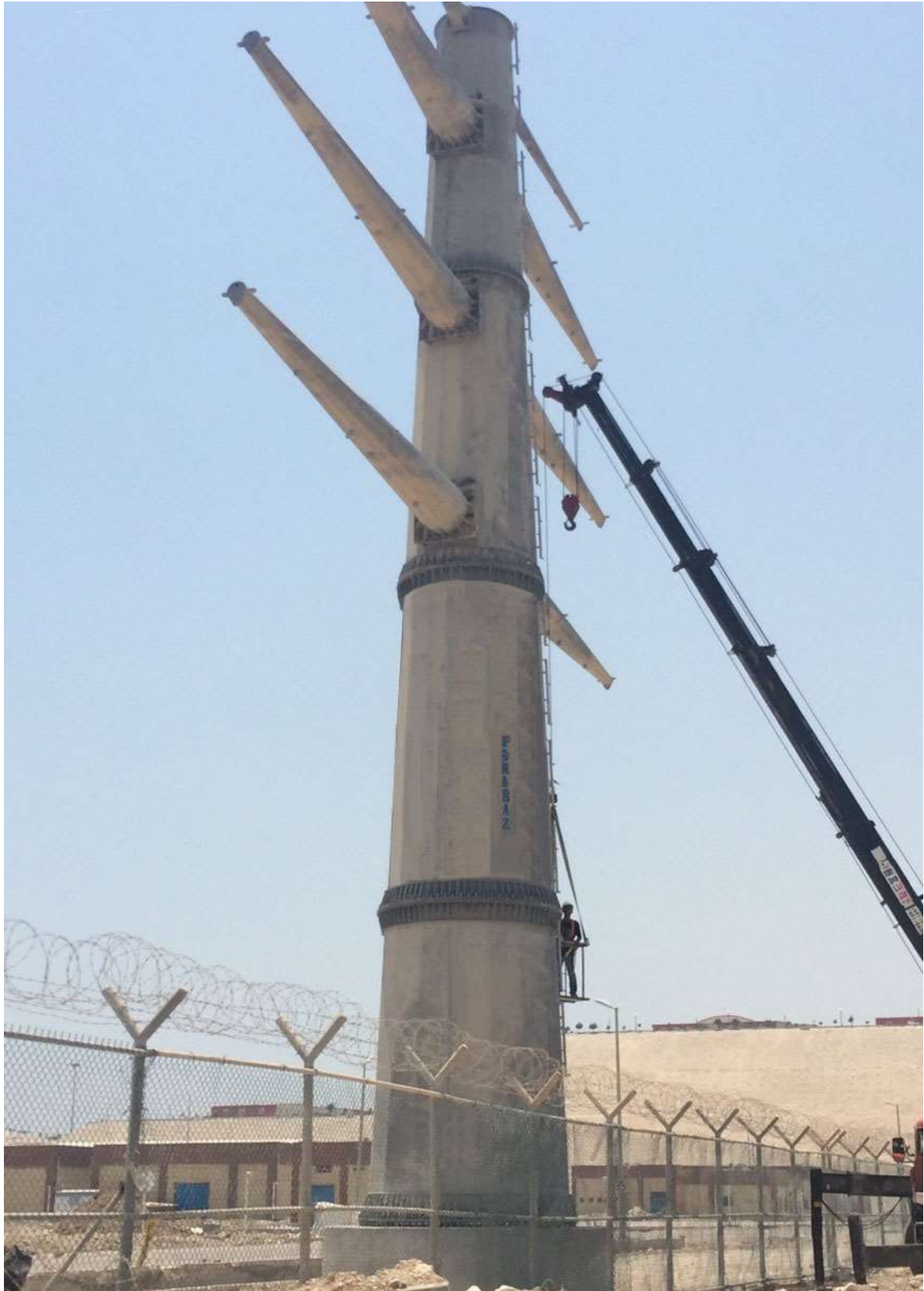
South Pars (Phase-1۳) ۱۳۲kv Four-Circuit Line under Construction
