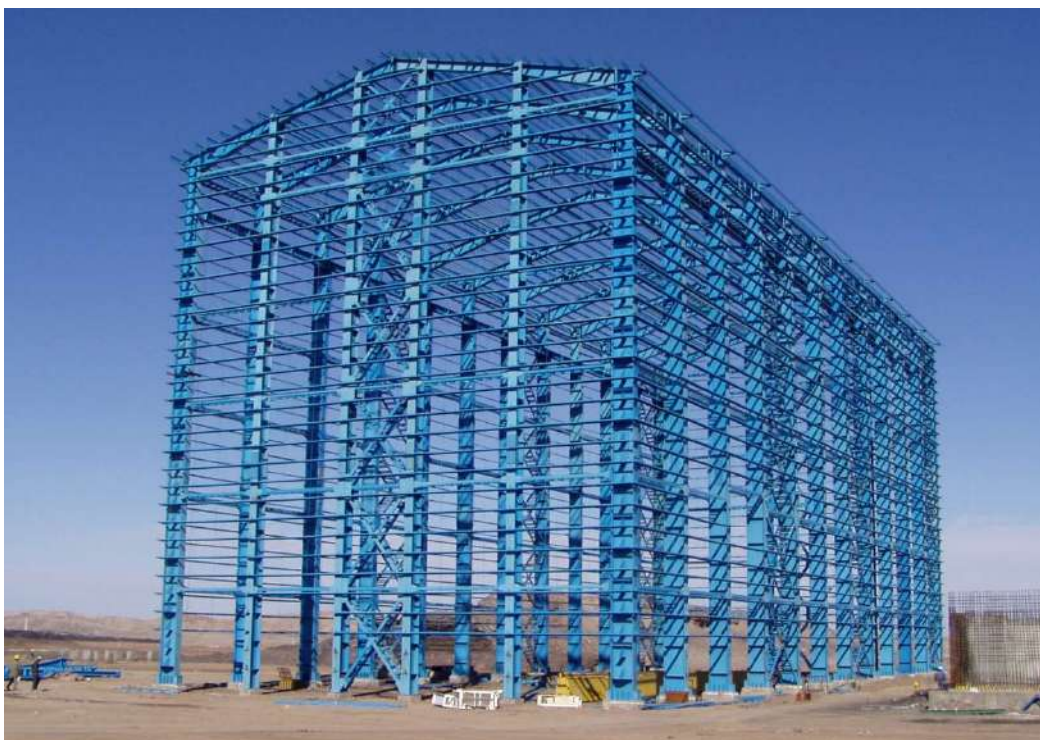
35m Structure for Tabas Coal Washing Project
