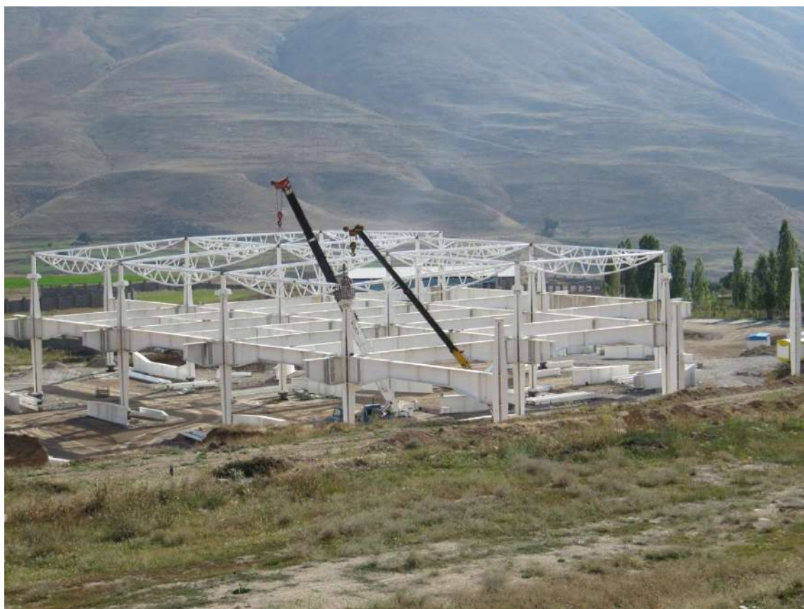
Vabel Factory Steel Structure while Erection
