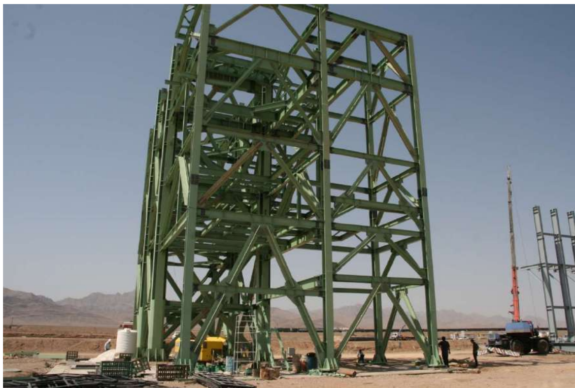
Ardekan Steel Complex Furnace Structure while Erection
