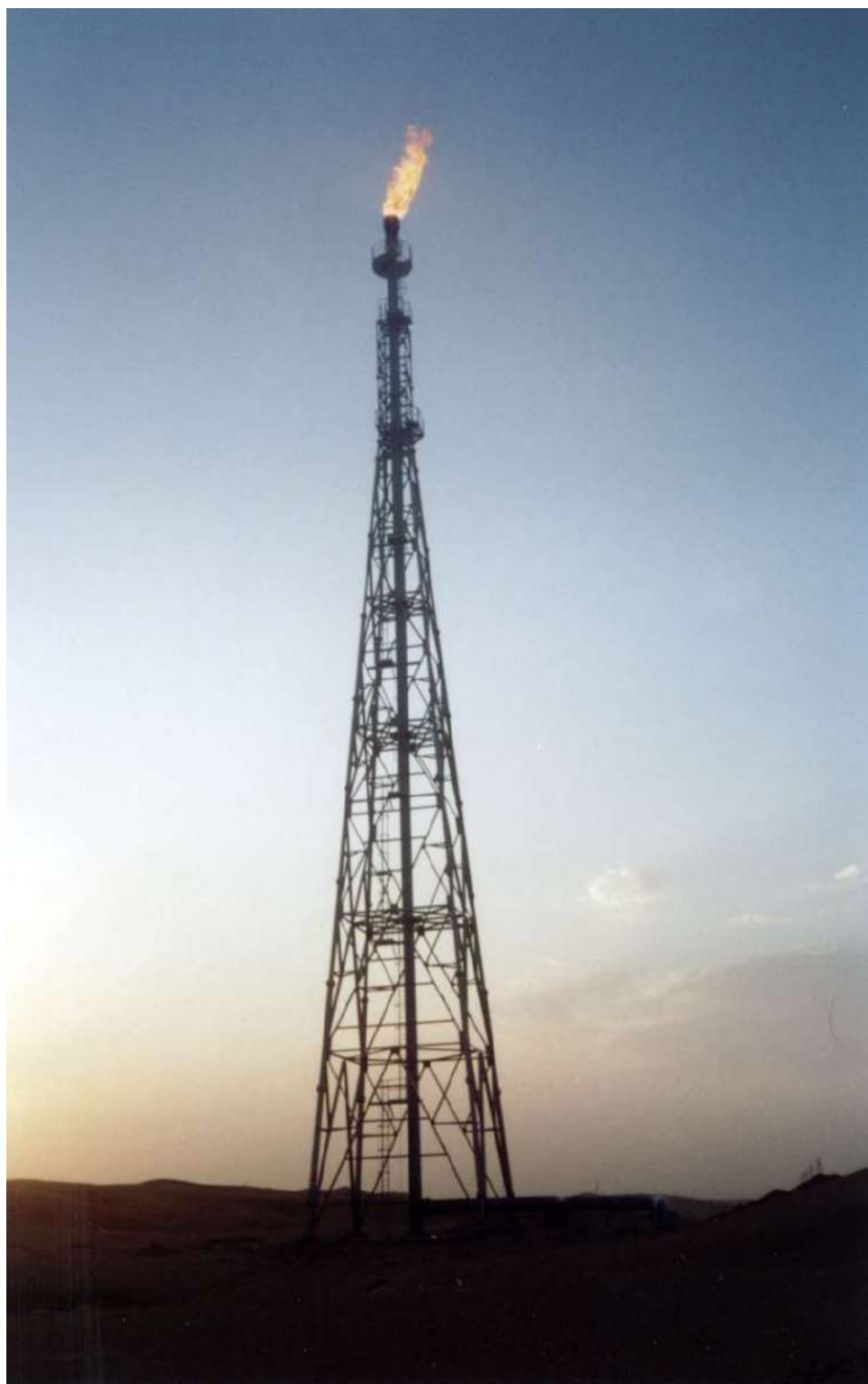
70m Derrick Tower in Korpedje, Turkmenistan
