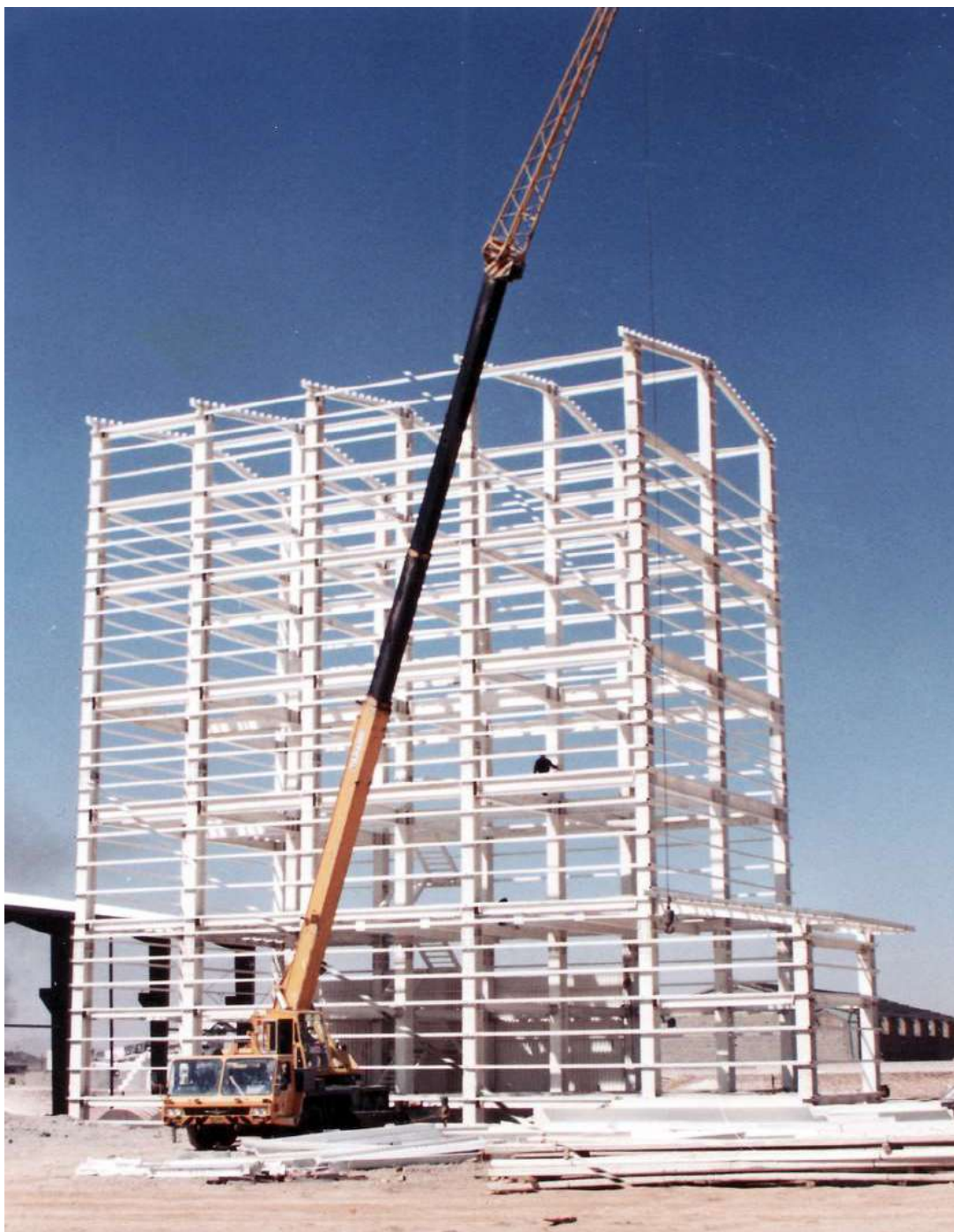
40m Structure of Isfahan Refractory Brick Factory
